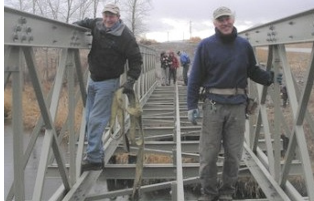
Lowering the bridge into place
